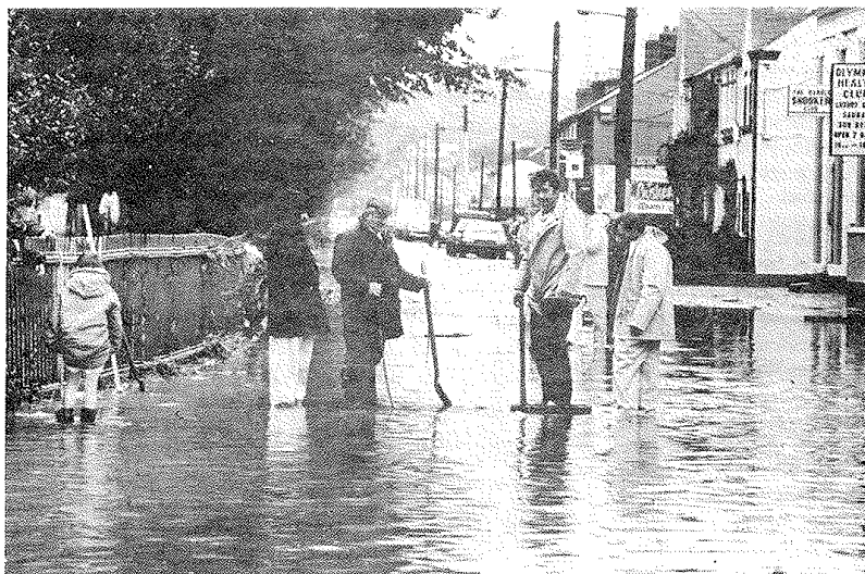
Bray after Hurricane Charley. Photograph courtesy Irish Times.
